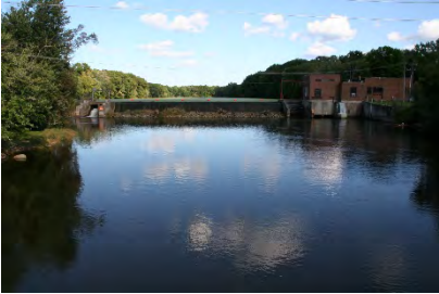
Smithville Dam (Smithville Park) |
